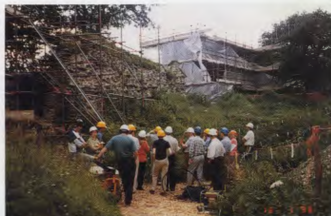
Members looking at works in progress; 'soft tops' re-established
