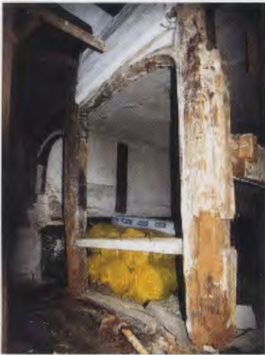
◀ Medieval shopfront after opening up
