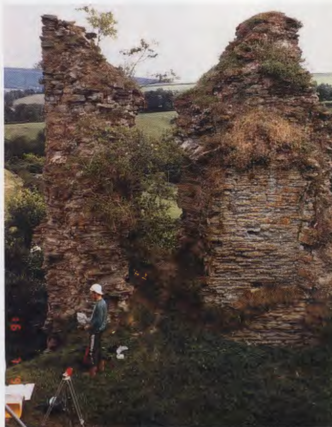
Section of ruin being recorded prior to consolidation works
