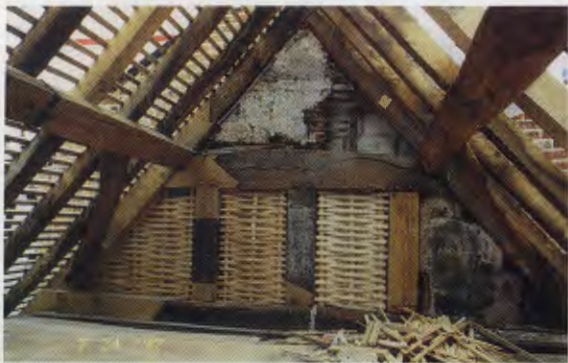
Medieval roof undergoing repair
