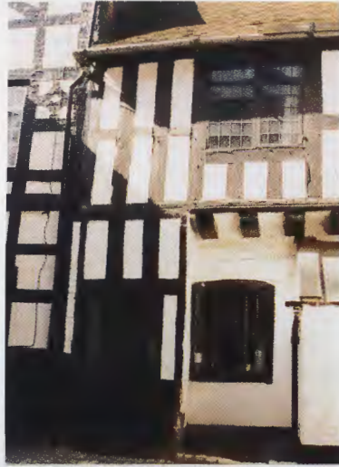
Medieval shopfront before opening up ▶
