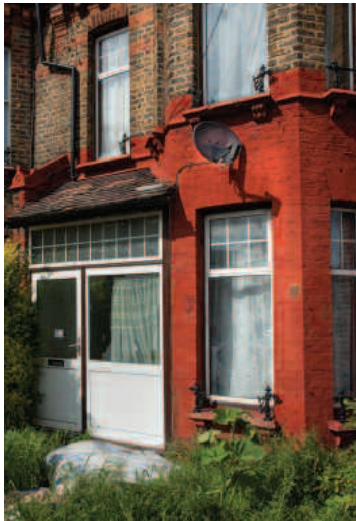
This late 19th century terraced house in the Noel Park Conservation Area in the London Borough of Haringey has had its historic character severely eroded by inappropriate uPVC windows and doors and unnecessary painting of part of the brickwork. A survey of estate agents carried out for English Heritage suggests that the value of properties that have been insensitively altered is likely to be lower than those that retain their original features intact
