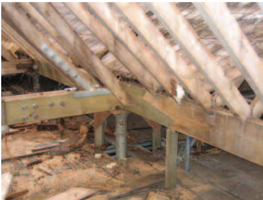
In situ repairs to valley beams and king post roof truss
