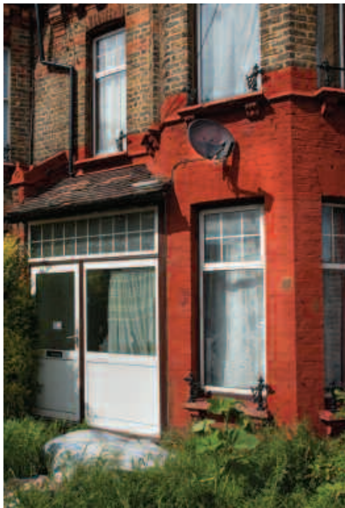
This late 19th century terraced house in the Noel Park Conservation Area in the London Borough of Haringey has had its historic character severely eroded by inappropriate uPVC windows and doors and unnecessary painting of part of the brickwork. A survey of estate agents carried out for English Heritage suggests that the value of properties that have been insensitively altered is likely to be lower than those that retain their original features intact
