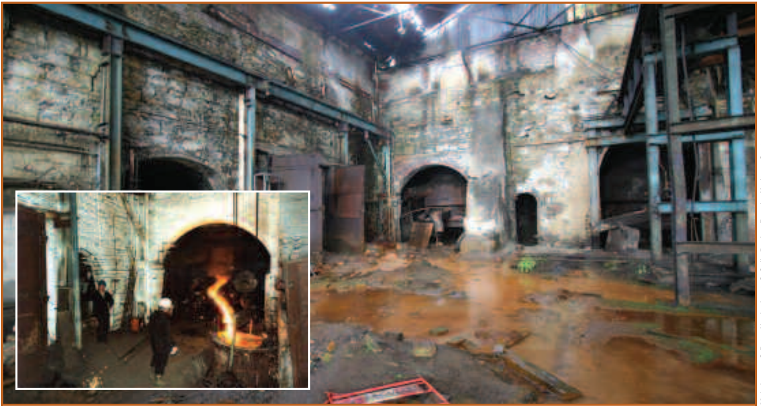
Part of the foundry in its present state and (inset) the furnace in use in the 20th century. Some elements of the original 18th century external walls survive.
