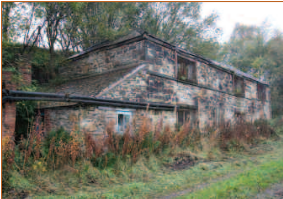
The agent's house (1794 or earlier); is a Grade II* listed building. This is a two-storey building situated on the south side of the heritage area. It has stone walls under a hipped slate roof and was extended at some stage at its west end, using materials of construction and design to match the original building.
